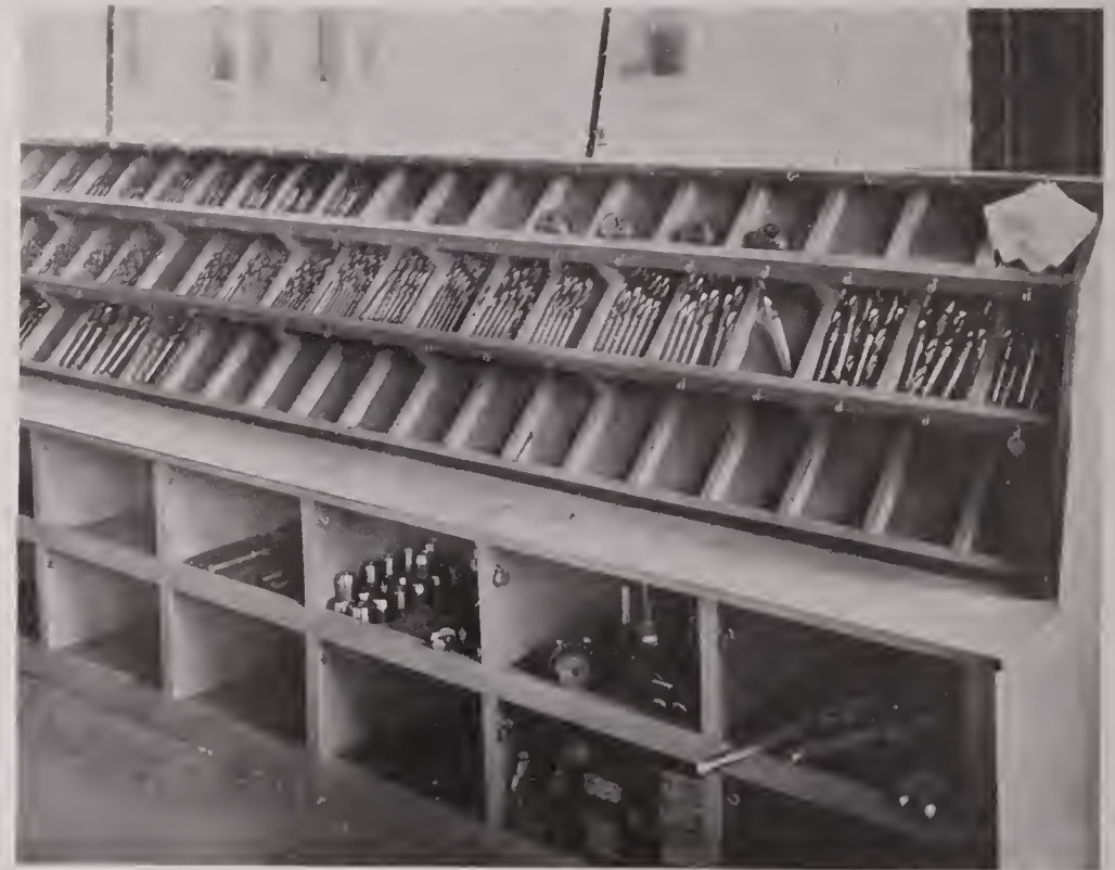
A SECTION OF THE TOOL CRIB
